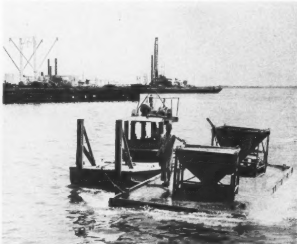
STURDY FLATBOAT chugs busily between dock structure and shore, delivering bucketsful of concrete and returning to mixer for refills. Workmen (below) smooth out concrete after it is poured on the deck.
